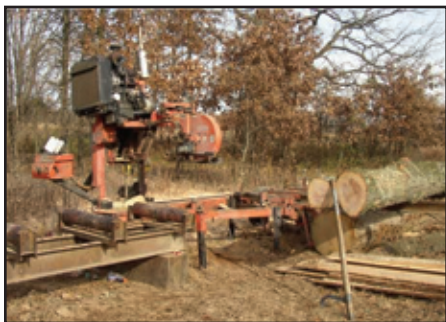
Crane mats are made from logs harvested and sawed on site.
